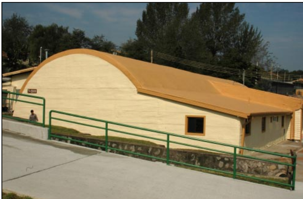
The Education Center at Camp Stanley nears completion and is slated to open in early November.
